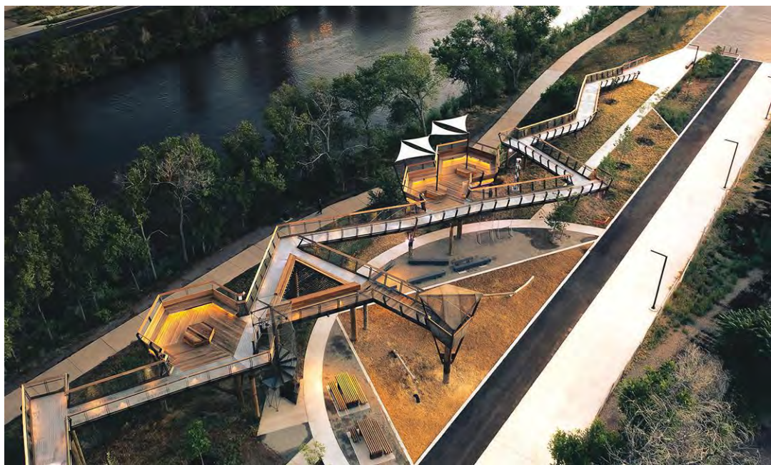
The promenade offers a road for bikes and pedestrians (top) alongside the accessible, elevated pathway (above). The net-covered spiral staircase is not required for entry or exit.
